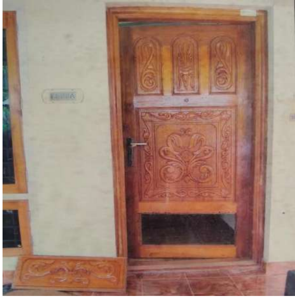
Fig 2: Door breaking (Type I)
