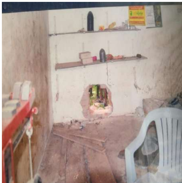
Fig 7: Theft by digging holes in the walls
