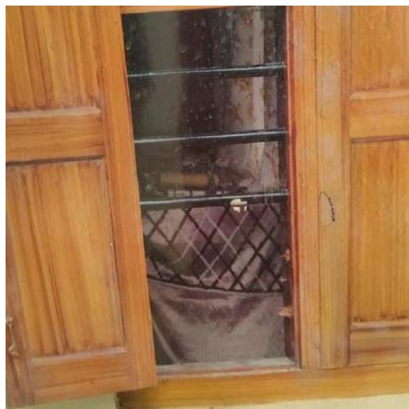
Fig 9: Break in through window grills
