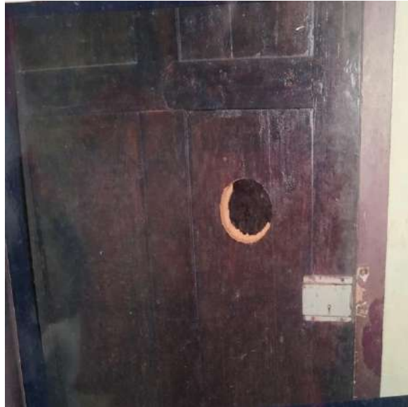
Fig 4: Door breaking (Type II)
