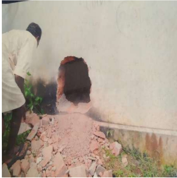
Fig 8: Hole on the wall; a view from outside the house
