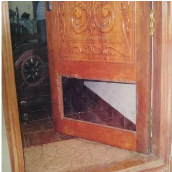
Fig 3: Close up view of door breaking
